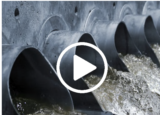
Industrial and storm drains treatment from oils, fats and petroleum products
